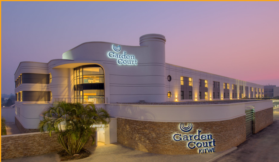
Side view of the Garden Court Hotel in Kitwe
