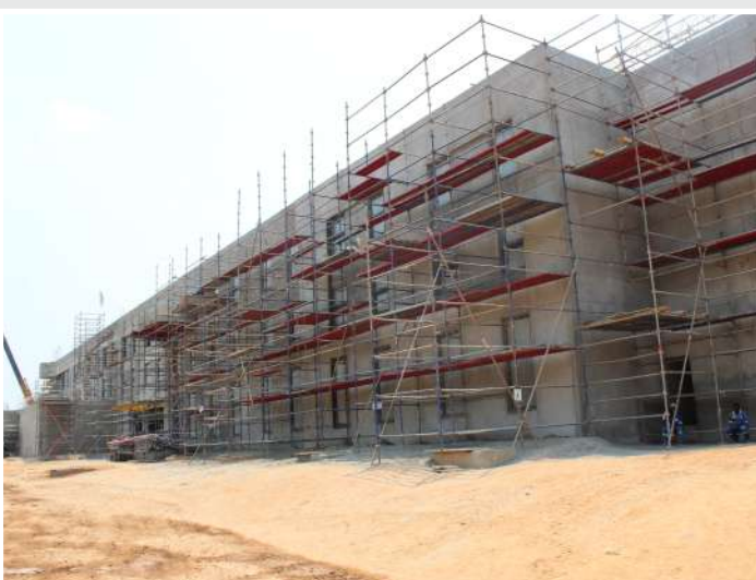
Side view of the ECL Mall in Kitwe being constructed .
